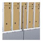
Insert splines to align reveals and ensure a clean, uniform finish. Then continue installing panels in any direction — left, right, or up — to keep crews moving without delay.
